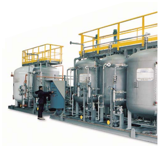
Sulphuric Acid, Biodispersant, Scale Inhibitor and Biocide Dosing Package
